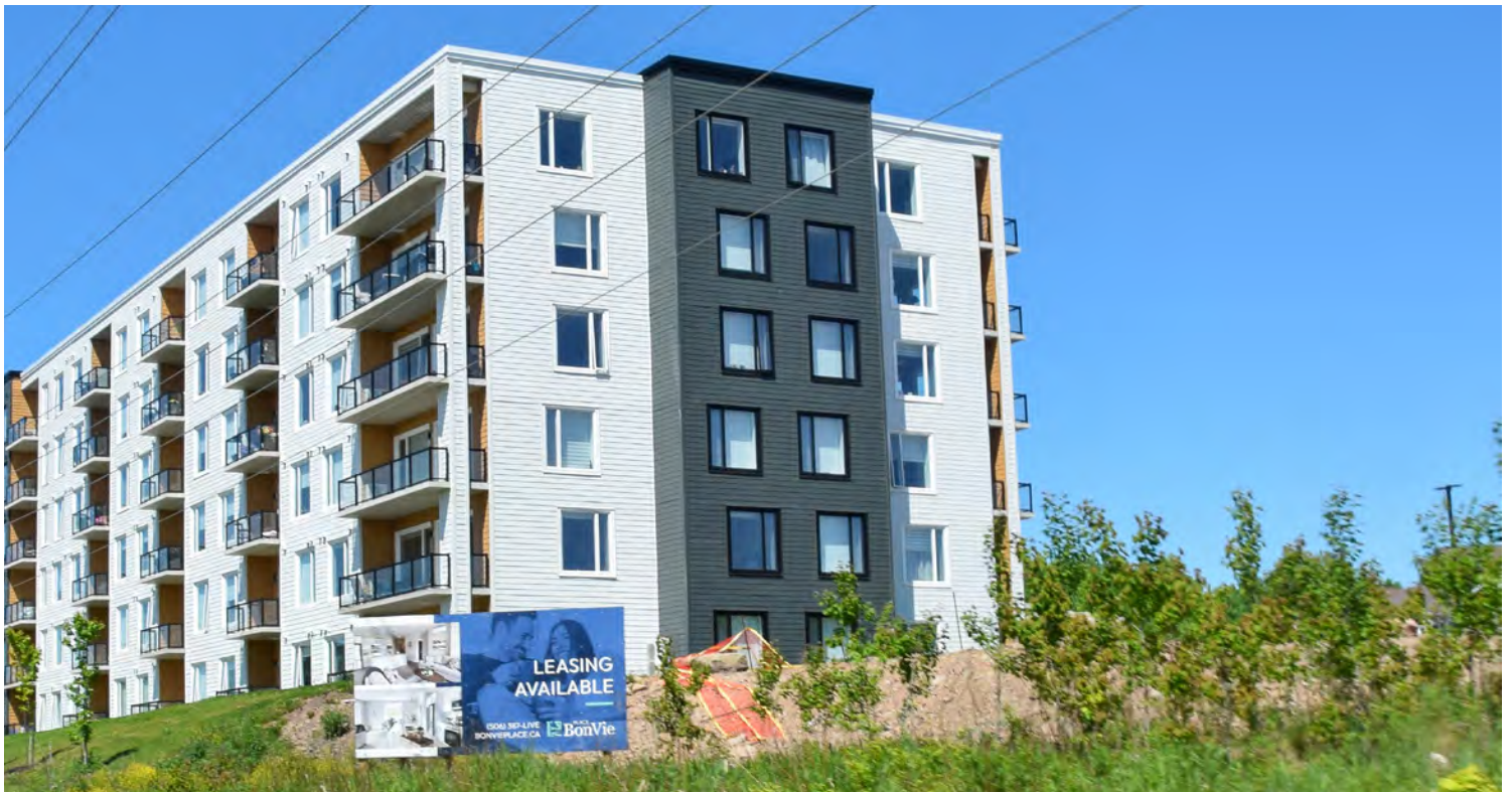
Figure 54: Recently constructed multi-unit dwelling on Dieppe Boulevard
