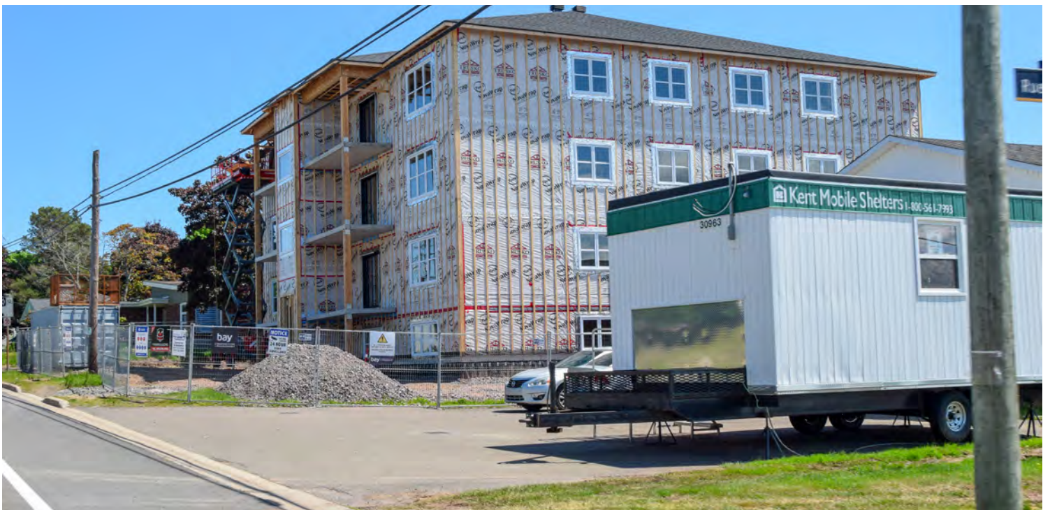
Figure 1: Construction site on Amirault Street.
