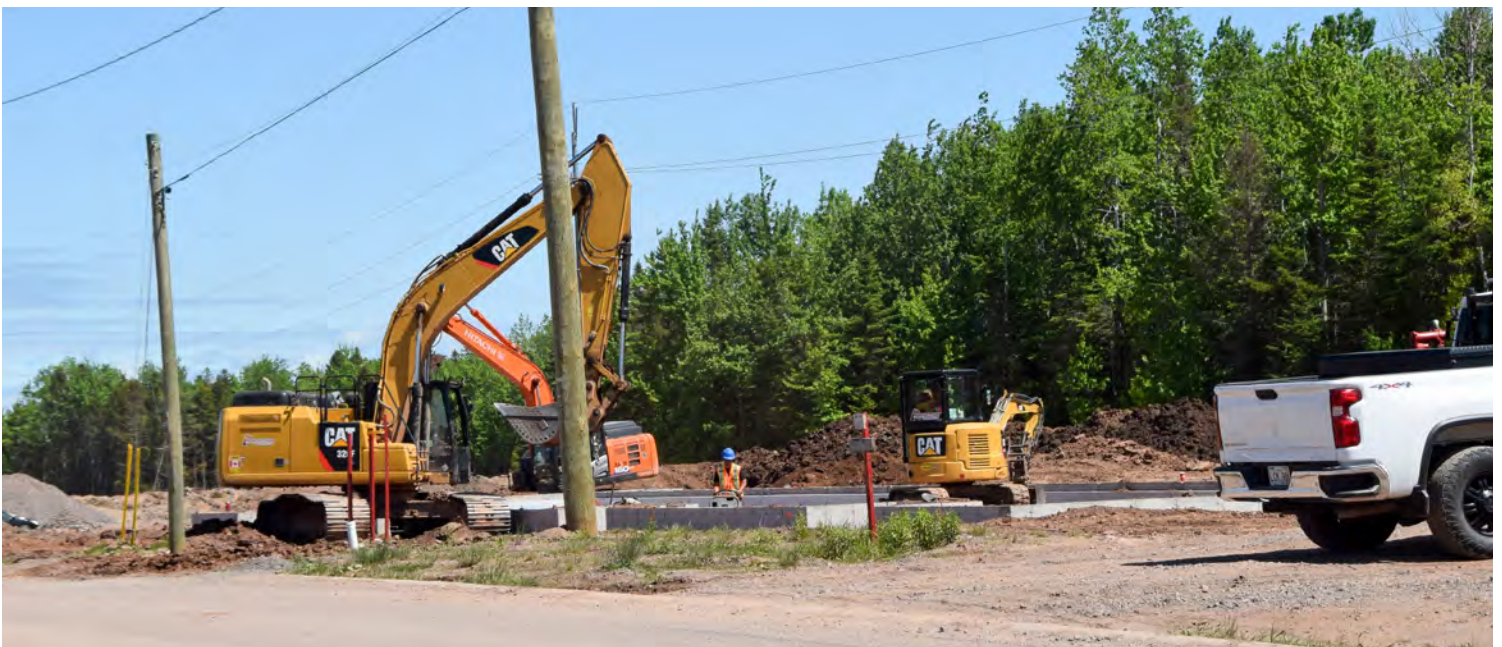
Figure 56: Home construction on Melanie Street
