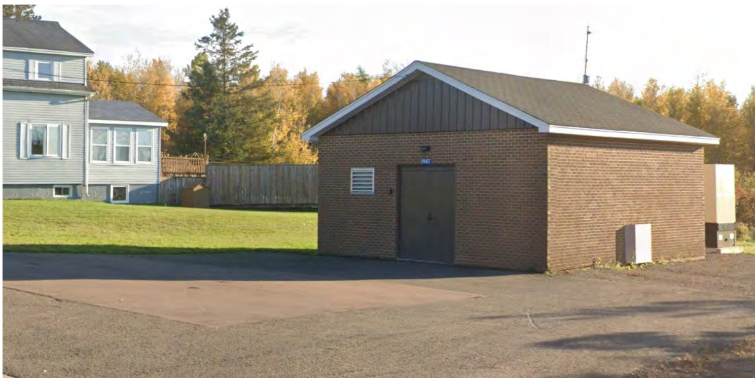
Figure 10: Booster station on Amirault Street (Image credit: Google Maps).
