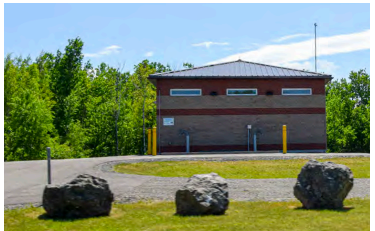
Figure 13: New Fox Creek sewage pumping station on Amirault Street
